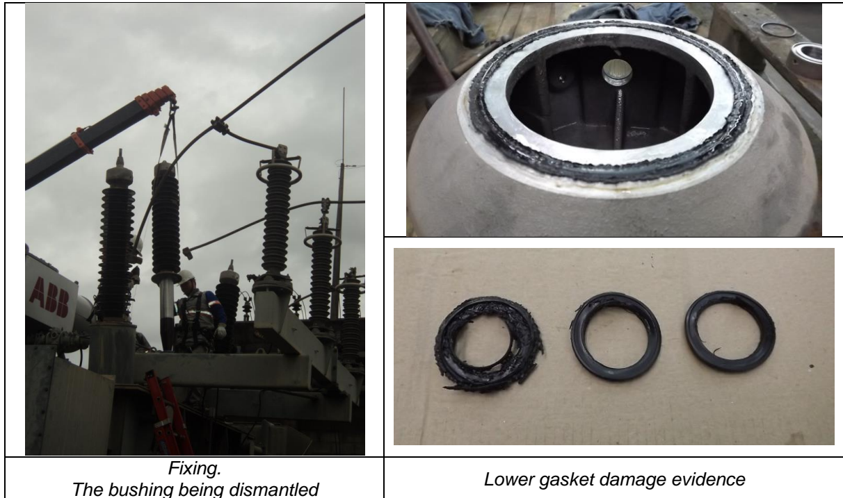
Figure 11. Physical state of the component with anomaly
